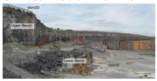
The quarry boundary is defined by a steel fence on a concrete plinth, which borders the Limestone pavement within the Lough Corrib cSAC. There is an average distance of approximately 1m between the edge of the fenceline plinth and the top of the upper quarry bench. **Figure 3.4** below shows a view of the western quarry wall from a distance, outlining the lower and upper bench and boundary fence.
